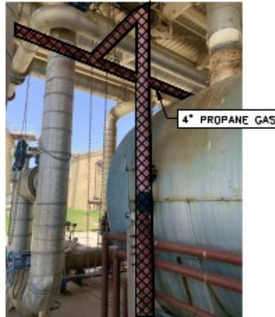
DESCRIPTION: BOILER #1 PROPANE GAS LINE (PG)
