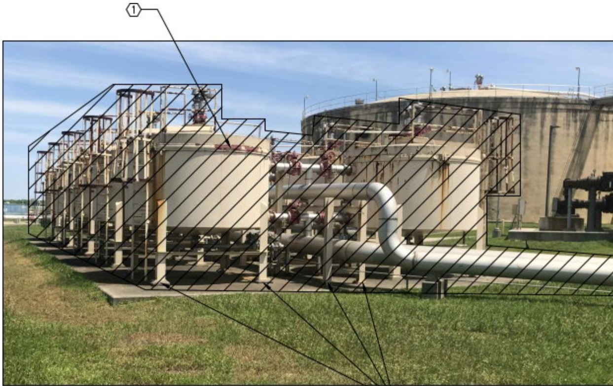
DESCRIPTION: VIEW OF IRON SPONGES FACING EAST.
